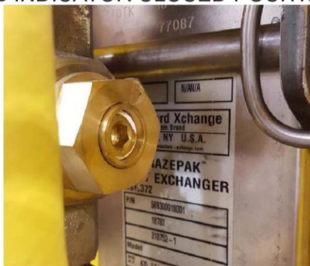
V3 INDICATOR CLOSED POSITION
