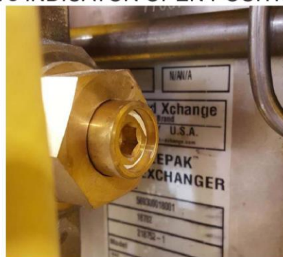
V3 INDICATOR OPEN POSITION
