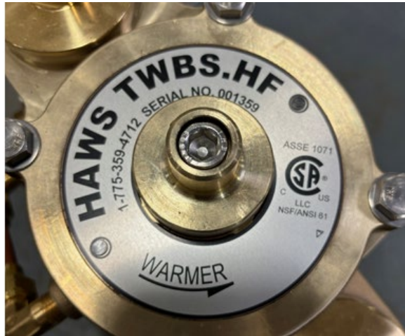
Figure 6. Blending Valve
