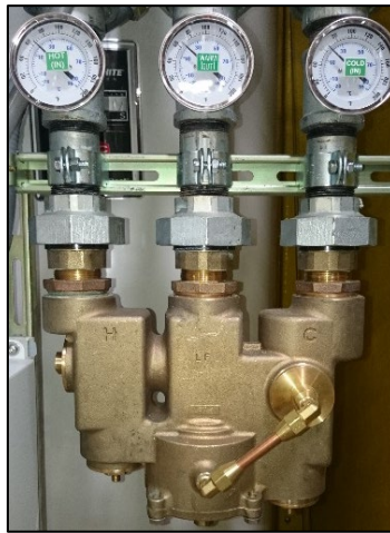
Figure 4. Blending Valve
