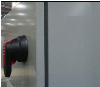
Figure 1. Disconnect Switch Junction Box
