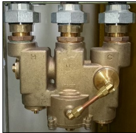
Figure 7. Blending Valve
