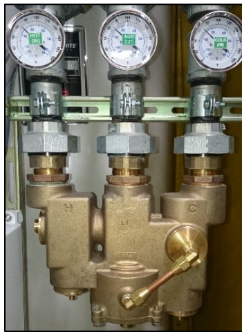
Figure 4. Blending Valve
