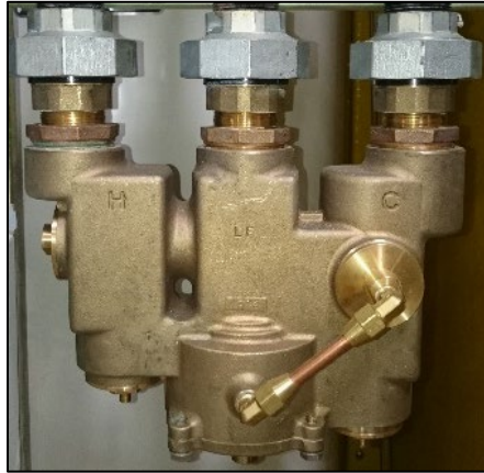
Figure 7. Blending Valve
