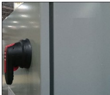
Figure 1. Disconnect Switch Junction Box
