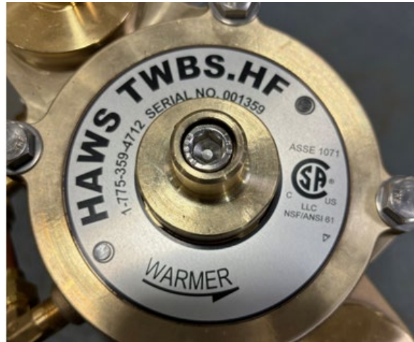
Figure 6. Blending Valve
