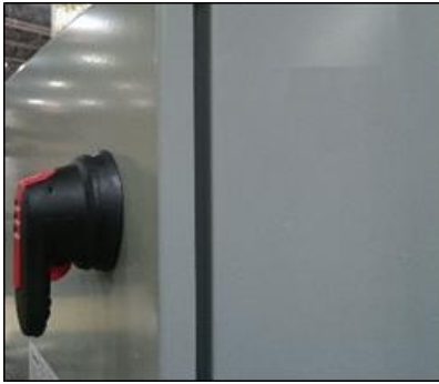
Figure 2. Disconnect Switch Junction Box
