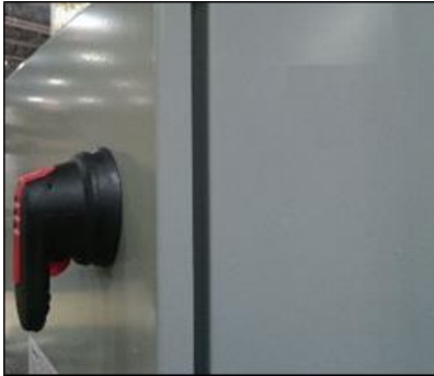
Figure 2. Disconnect Switch Junction Box
