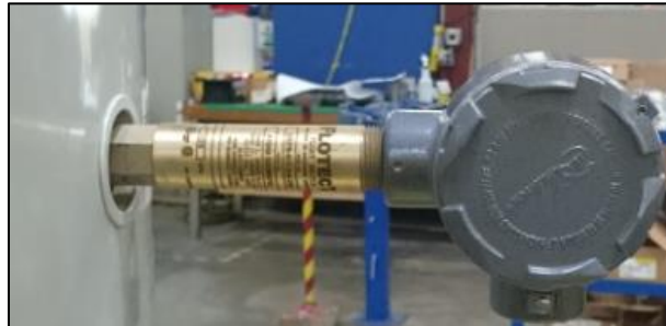
Figure 6. Level Switch
