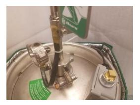
**STEP 7:** Attach junction box to tank handle with supplied cable tie.
