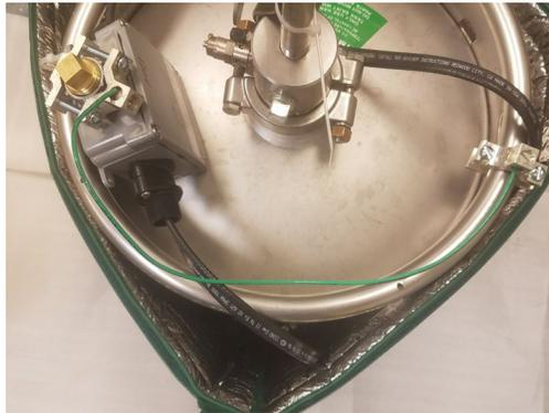
**STEP 8:** Attach conical top blanket with Velcro closures. Align the seam of the top blanket with the push flag. The electrical cord may exit across the Velcro seam at any location.
