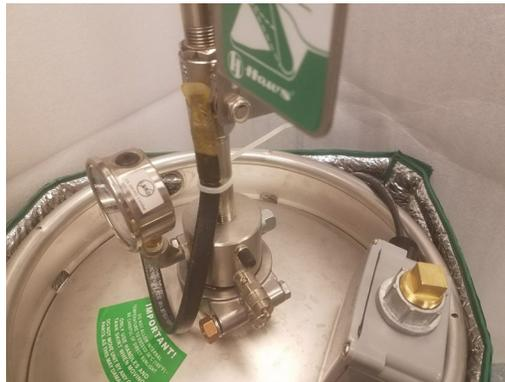
**STEP 6:** Attach junction box to tank handle with cable tie.
